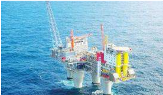
Power from shore/ Ship to Shore
