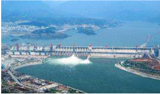
Connecting remote generation
